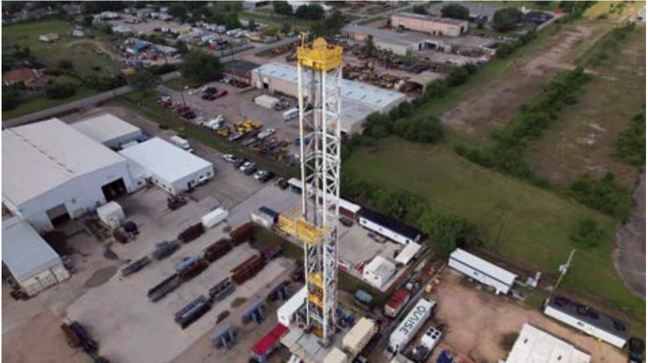
FIGURE 4.4 Drone image of the setup for the first demonstration of Quaise Energy's novel drilling technique on a full-scale oil rig
