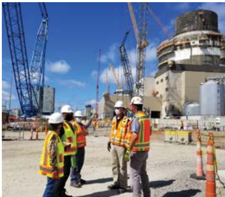
FIGURE 4.3 Vogtle Unit 3 under construction in October 2020
